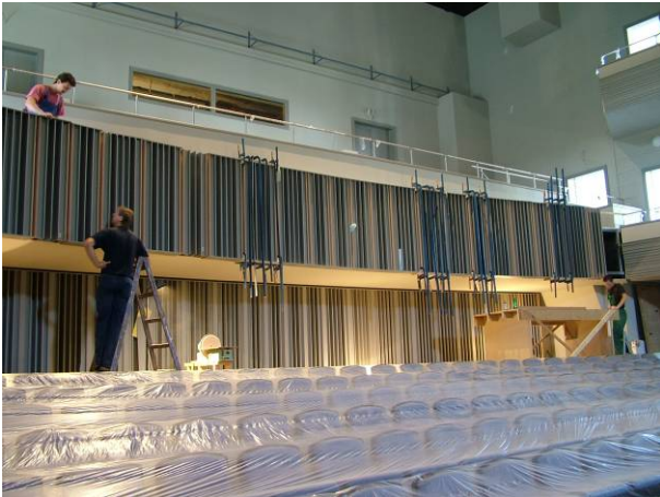
Figure 20. Assembly of the QRD diffusers on the rear wall
