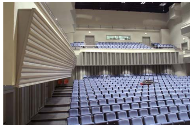
Figure 23. View at the interior acoustic design, detail of the position of the reflective and scattering structures on the side balconies
